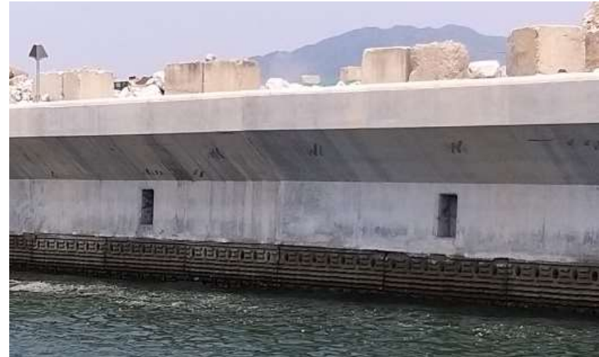
General View of Vertical Eco-shoreline
